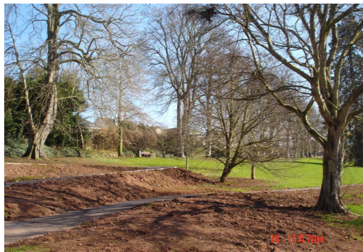
The planting areas run alongside sections of the pathway. At present they are bare earth.
